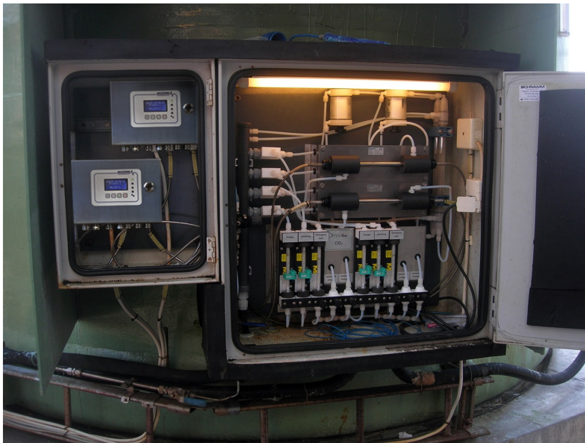
Kemtrak DCP007 process photometer with 200mm optical path length PTFE 25%C - titanium measurement cell and extractive gas sampling system installed at the outlet
